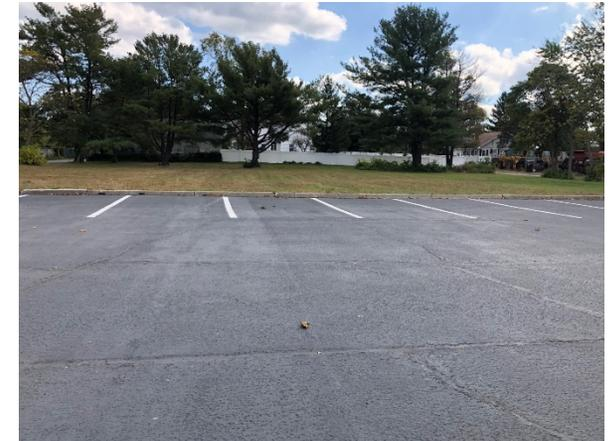
Parking spaces in the parking lot to the east of the building can be converted to porous pavement to capture and infiltrate stormwater runoff from the parking lot. Rain gardens can be installed in the turfgrass at the entrance and rear of the building to capture, treat, and infiltrate stormwater runoff from the roof. A preliminary soil assessment suggests that more soil testing would be required before determining the soil's suitability for green infrastructure.
