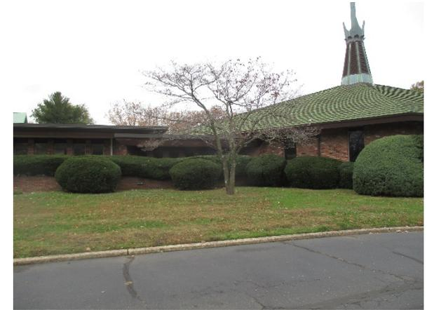
Parking spaces in the parking lot to the south of the building can be converted to porous pavement to capture and infiltrate stormwater runoff from the parking lot. Rain gardens can be installed in the turfgrass areas around the building and near a section of parking spaces to capture, treat, and infiltrate stormwater runoff from the roof and parking lot. A preliminary soil assessment suggests that the soils have suitable drainage characteristics for green infrastructure.
