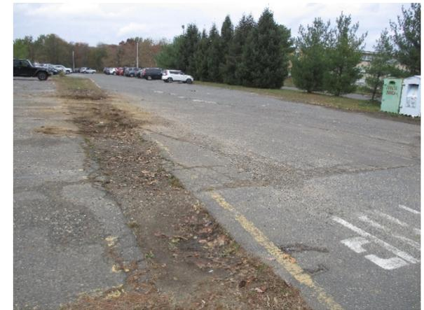
A row of parking spaces to the north of the main building can be converted to porous pavement to capture and infiltrate stormwater runoff from the parking lot and roof. Rain gardens can be installed at various locations to capture, treat, and infiltrate stormwater runoff from the roof. A preliminary soil assessment suggests that the soils have suitable drainage characteristics for green infrastructure.
