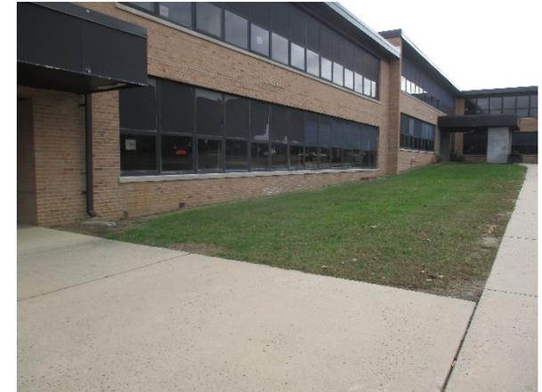
Parking spaces in the parking lot to the north of the building can be converted to porous pavement to capture and infiltrate stormwater runoff from the parking lot. Rain gardens can be installed at several locations to capture, treat, and infiltrate stormwater runoff from the rooftops. A preliminary soil assessment suggests that the soils have suitable drainage characteristics for green infrastructure.
